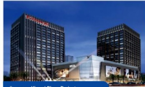
Jiangmen Kinwai Plaza Project
