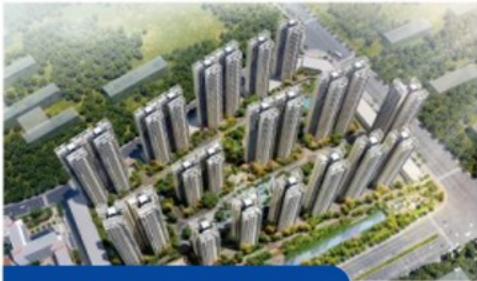
Zhenjiang China Resources Taoyuanli Project
