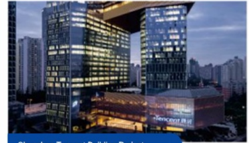
Shenzhen Tencent Building Project
