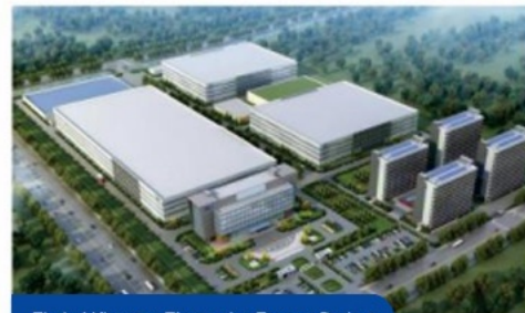
Zhuhai Kinwong Electronics Factory Project
