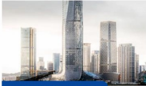
Hengqin International Finance Center Project
