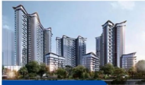
Poly Xiutai Tianjun Project
