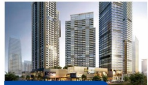
Shenzhen Hansen Yuehai City Project
